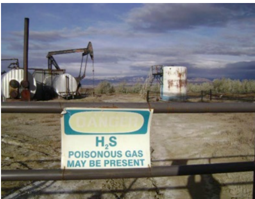
Figure 2: Current regulations merely require posting signs warning of the H 2 S hazard on the wells' fencelines. These signs themselves are corroding.
